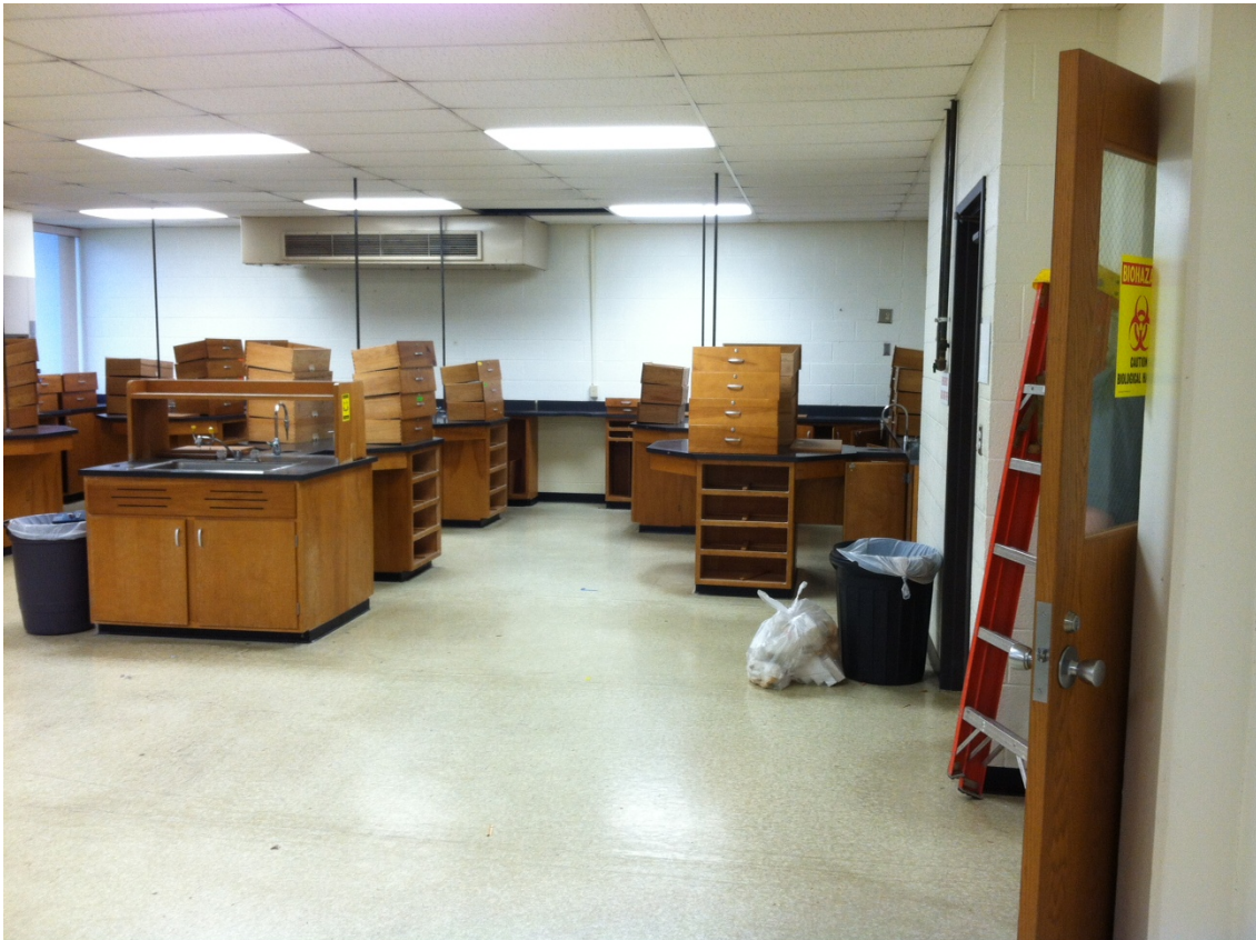
Stoltz Room 9 prior to demo
