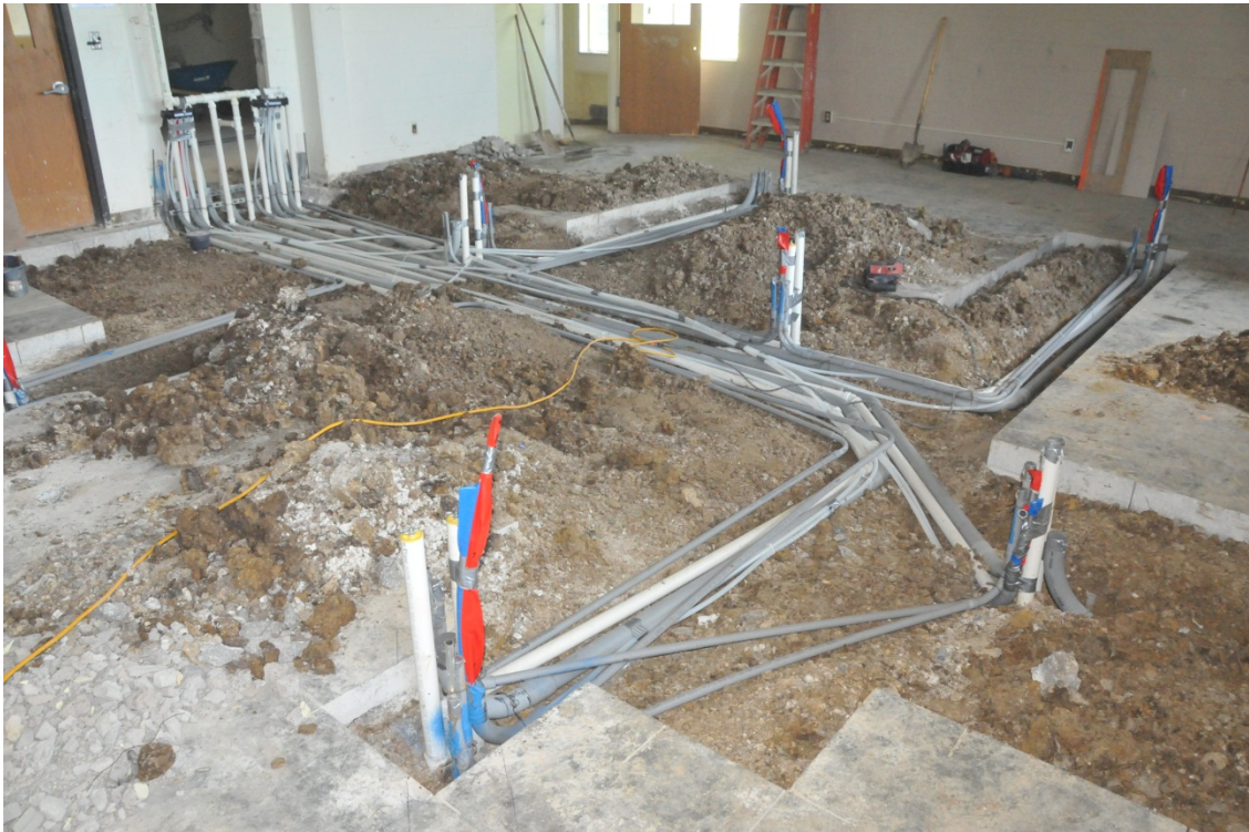
Stoltz Room 9 plumbing/electrical rough-in
