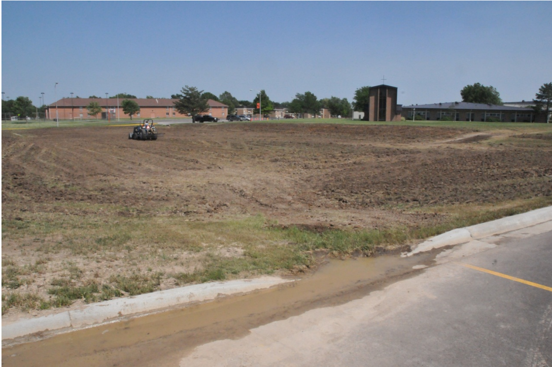
North Detention Basin re-grade and re-seed
