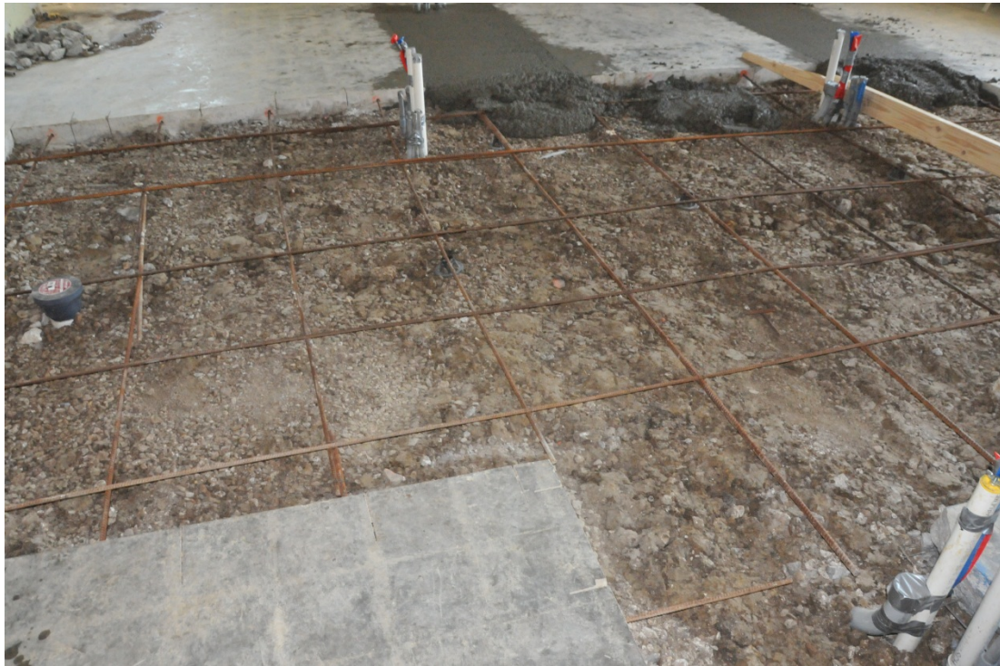
Stoltz Room 9 prior ready for concrete
