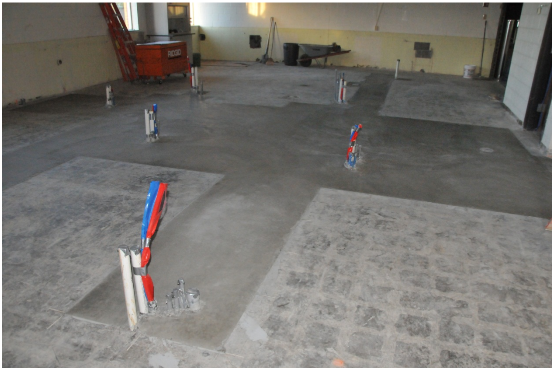
Stoltz Room 9 after concrete
